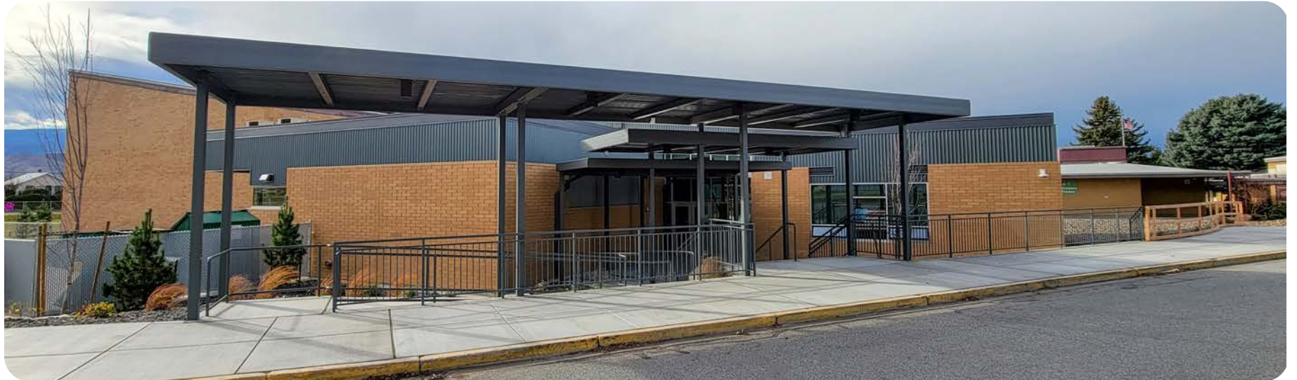
The outside of Cascade Elementary's new cafeteria. The Phase 1 Capital Levy funded new cafeterias and kitchens at four elementary schools.
